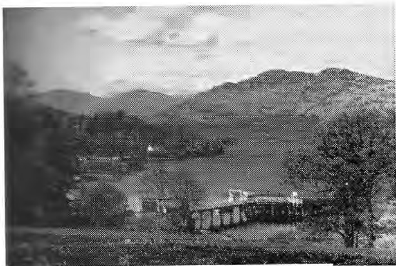
Plate 8. TARBET PIER, LOCH LOMOND
